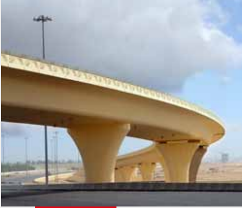
AL MAFRAQ INTERCHANGE BRIDGE
